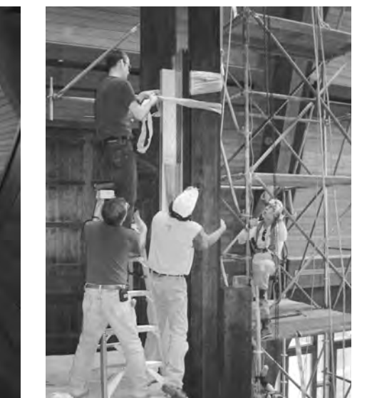
Hoisting and installing façade posts
