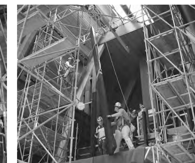
Lifting façade posts with scaffolding and hoist
