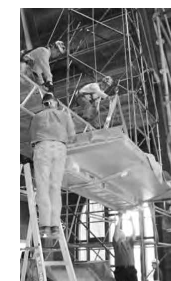
Lifting a windchest
