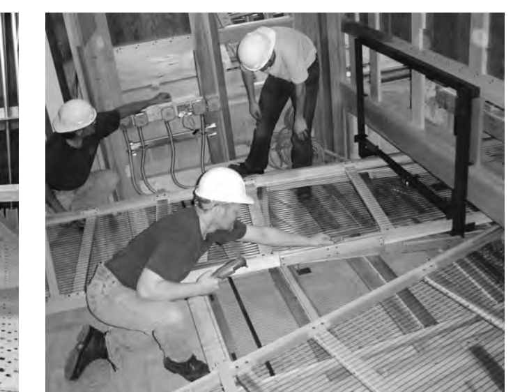
Installing splayed key action from console (at right) to case
