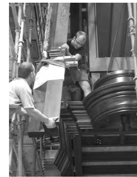
Hoisting front façade post, right case
