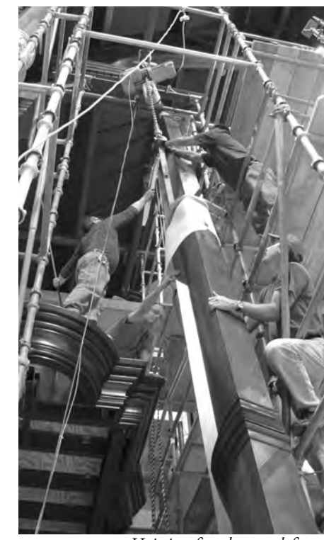
Hoisting façade post, left case
