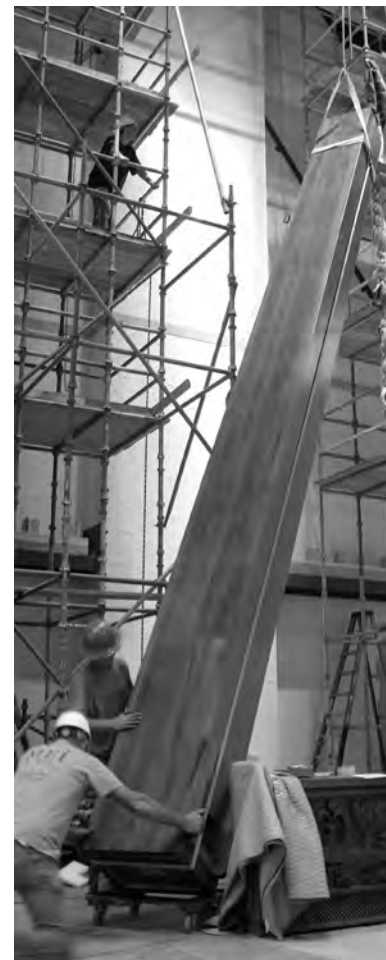
Hoisting 32' C of the Open Diapason
