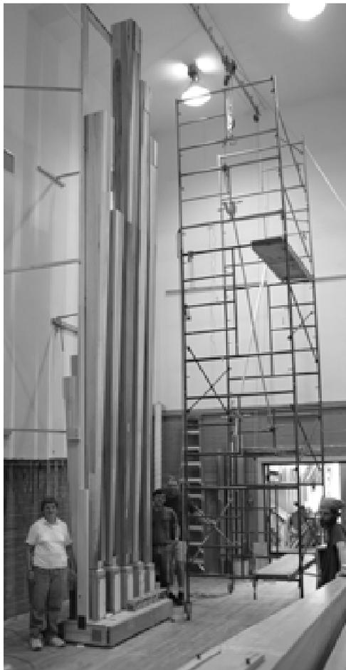
*Racking the 32' reed: upper halves of 64' A# and 32' C are too tall for the erecting room*
