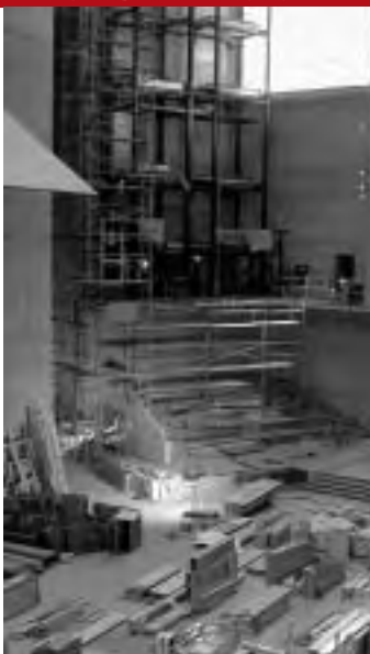
A myriad of parts awaits installation
