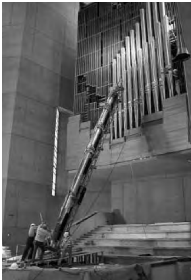
Using a support cradle, 32' C# is muscled into vertical position
