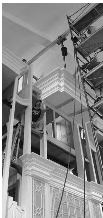
A tower top is hoisted
