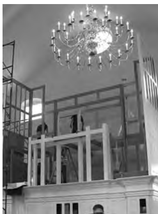
Partially assembled casework
