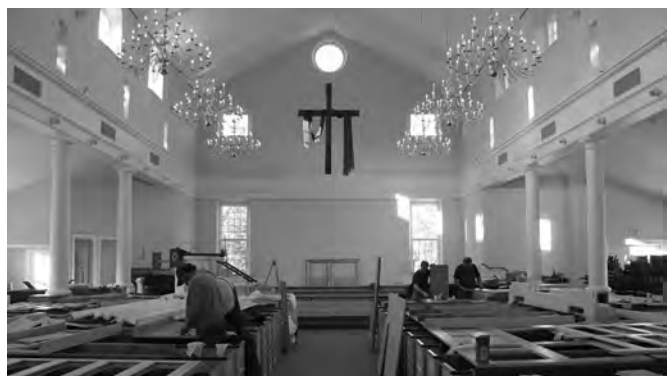
The chapel as work begins
