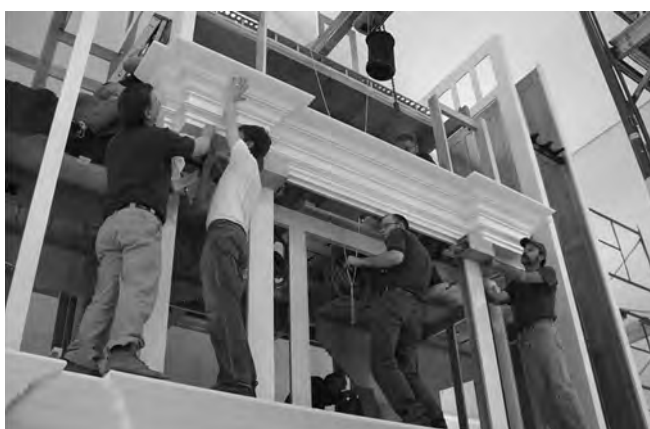
Installing the Great impost molding
