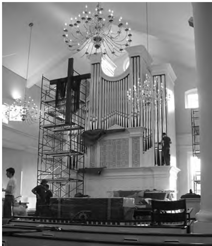
The fully assembled case before pipe shades are installed
