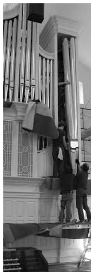
Installing the 16' Principal
